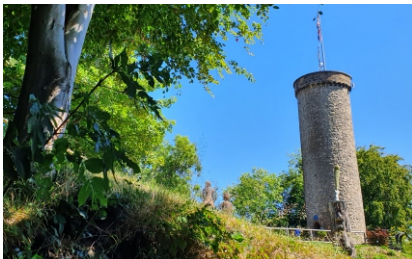
The Victoria Prospect Tower
